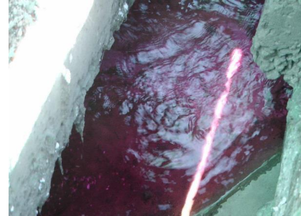
Purple dye used to trace storm water outlet
