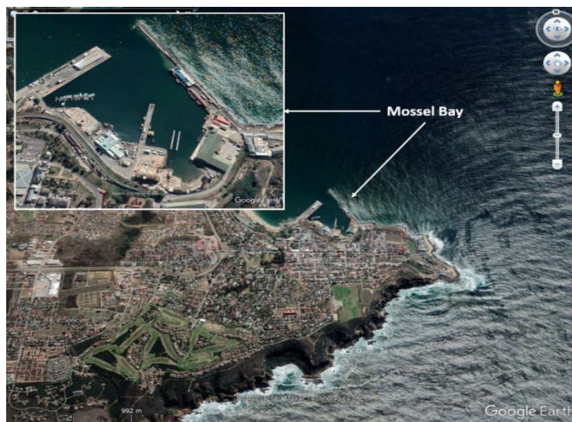
Figure 15 Port of Mossel Bay Aerial Photograph.
