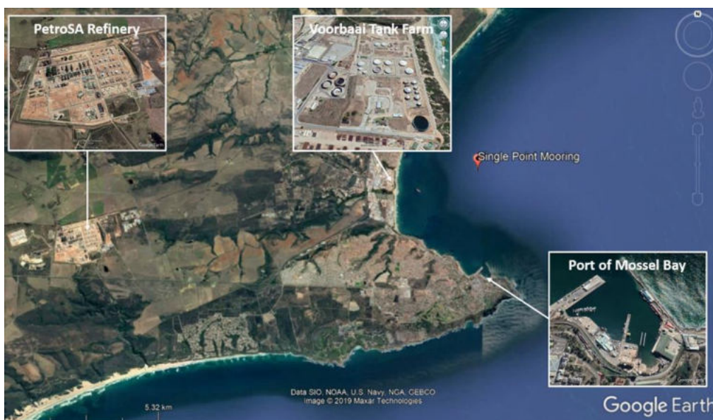
Figure 16 Port of Mossel Bay Aerial Photograph.
