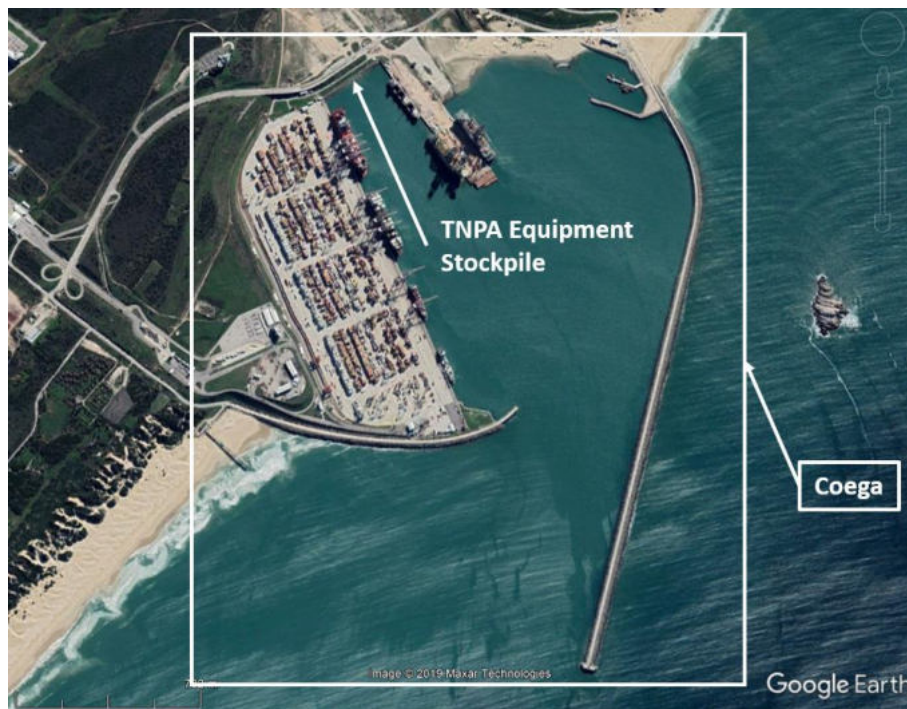
Figure 23 Port of Ngqura Aerial Photograph showing the TNPA Stockpile location.
