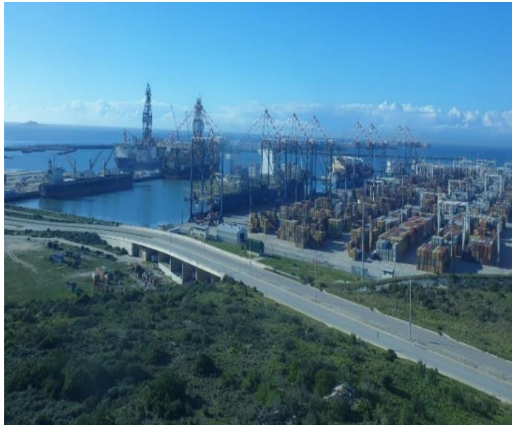
Figure 9 Ngqura (Coega) Terminal.
