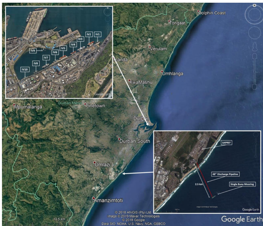
Figure 12 SBM, Pipeline, Refinery and Island View berths.
