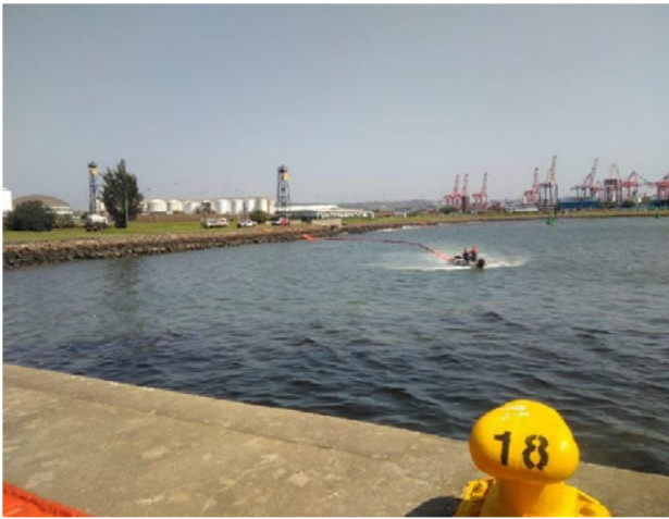
Service Provider deploying fence boom at
