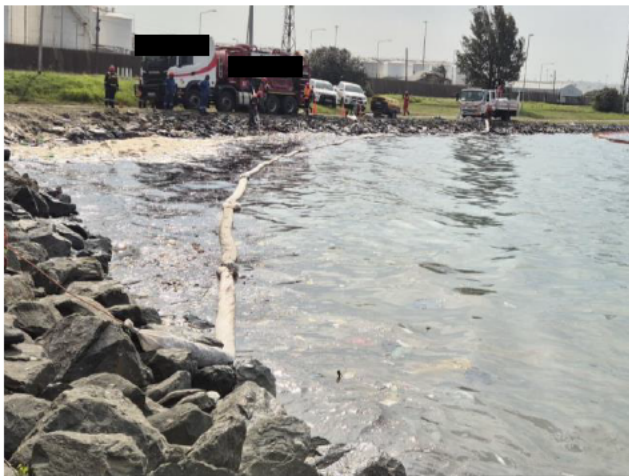
Service Provider Super Sucker recovering product at Causeway Corner
