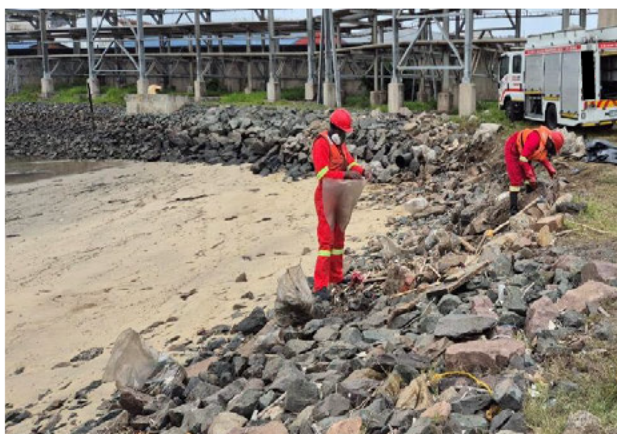
Service Provider removing debris from Causeway Corner
