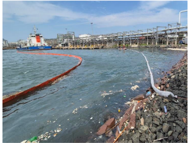
Service Provider deploying sausage boom at causeway
