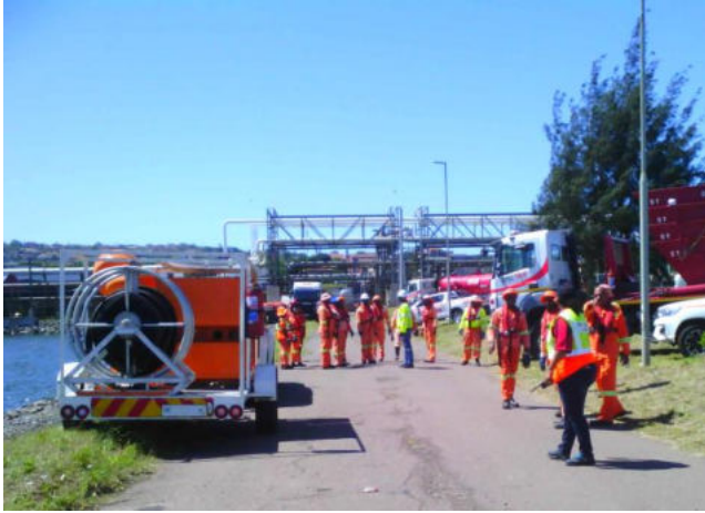
Staging area established at Causeway Road
