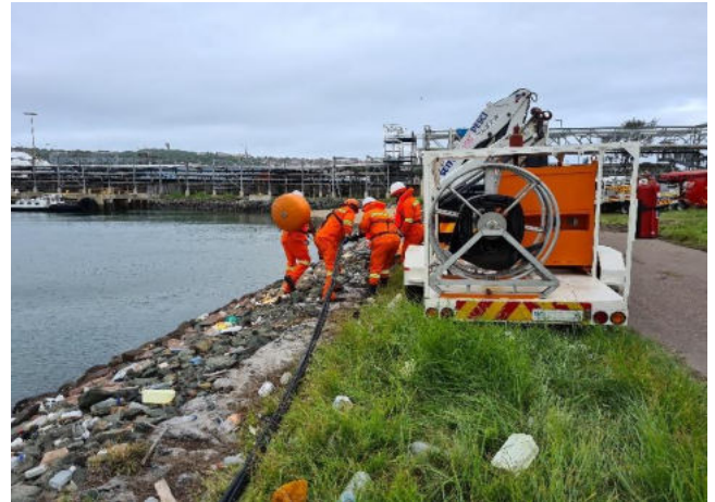
Staged equipment to be deployed
