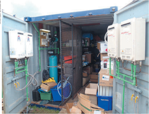
Massey University's mobile wash-water facilities include water heaters and a water softening system installed in an intermodal container for easy transportation.
