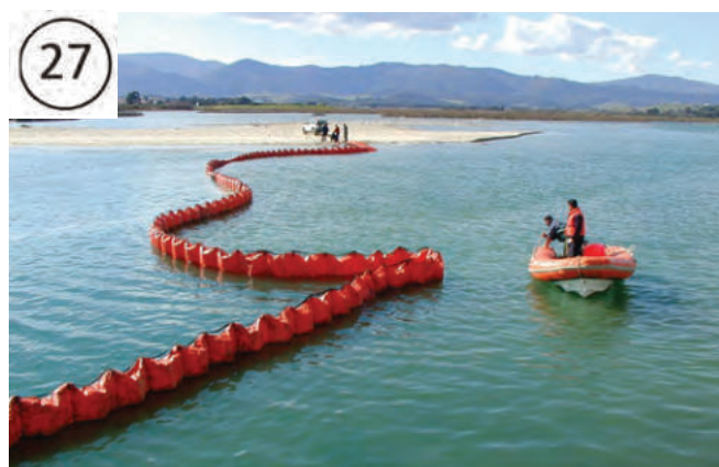
Figure 5: Boom deployment site near the river mouth. The boom is being set to deflect oil to a collection point with good access on the shore.
