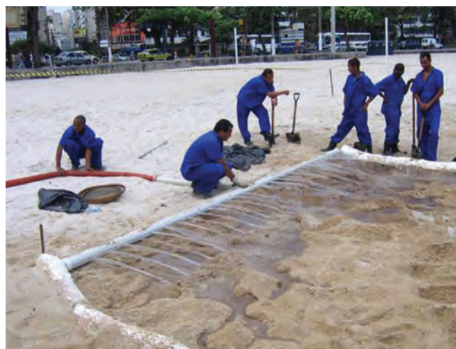
▲ Figure 1: Cleaning of oiled sand in-situ by low pressure flushing, with sorbent boom deployed appropriately to capture released oil.
