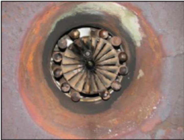
Photo 3 – Minor Refractor Repair
