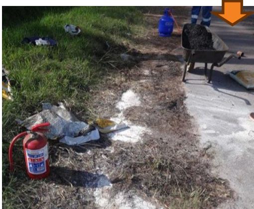
Picture 1: Wheelbarrow used to heat up Asphalt
