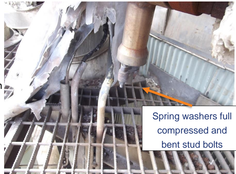
Fire damage to Instrumentation lines and fire blanket at 11-KV1030D
