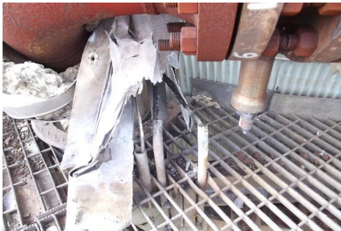
Fire damage to Instrumentation lines and fire blanket at 11-KV1030D
