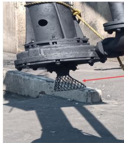
86PC-510 B after the pump was removed from CB-502 sump
