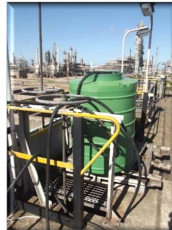
Temp Mixing Tank / MOCA in place.
