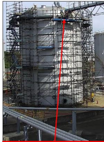
Two employees modifying scaffolding
