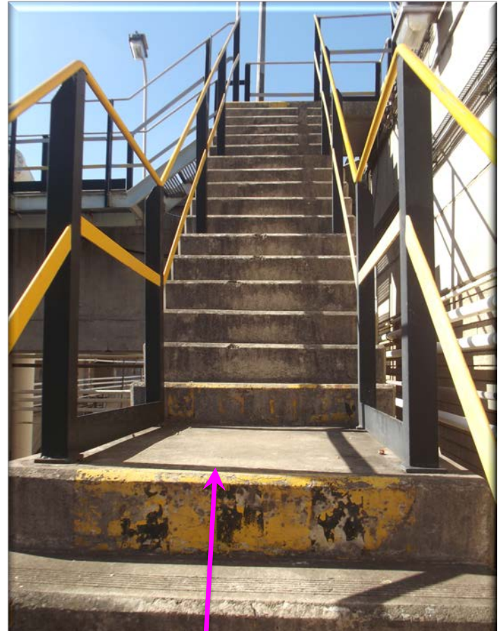
Staircase with 33 steps at Flocculation Channels
