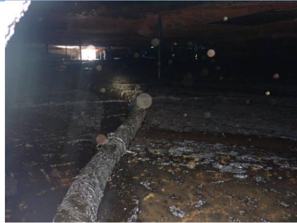
1: 6-Inch Suction Rubber Hoses that was lifted.
