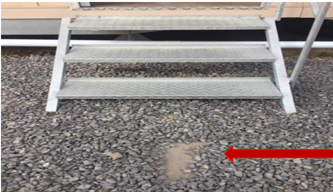
The employee slipped in the graveled area leading to Knee injury.
