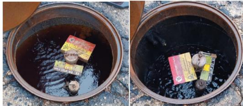
Tank 1&2 manholes filled with ULP93 and water
