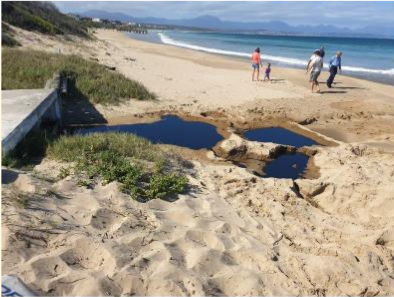
Photograph 1: Condensate spill at beach
