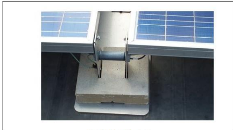
Fig. 2.1.1.11a. Slotted pedestal
